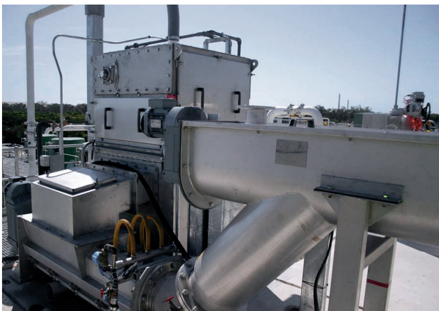
Centre-Flo directly discharging to Noggerath® Screening Wash Press NWP
