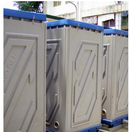
BioGill bioreactors were retrofitted to an existing STP in Manila to improve BOD reduction and reduce energy consumption.
