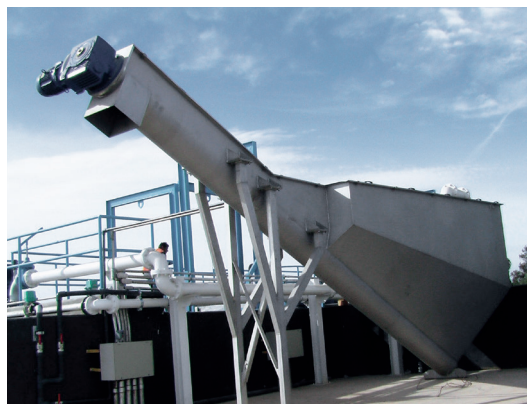
Installation for dewatering of grit trap settlings GS 130
